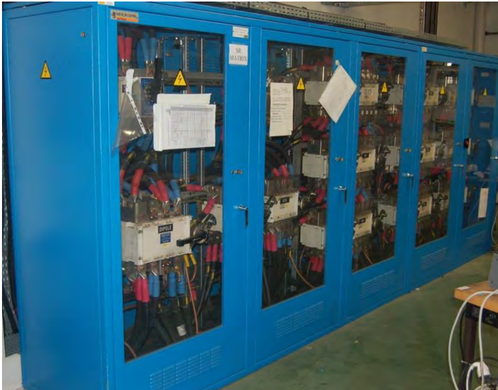
Figure 4.7: Switching Matrix serving the family power supplies.
