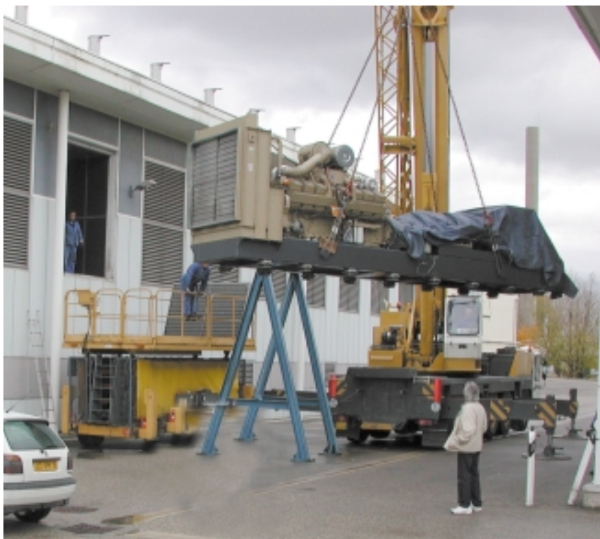
Fig. 2: Extraction of a beam support from the HQPS building.
