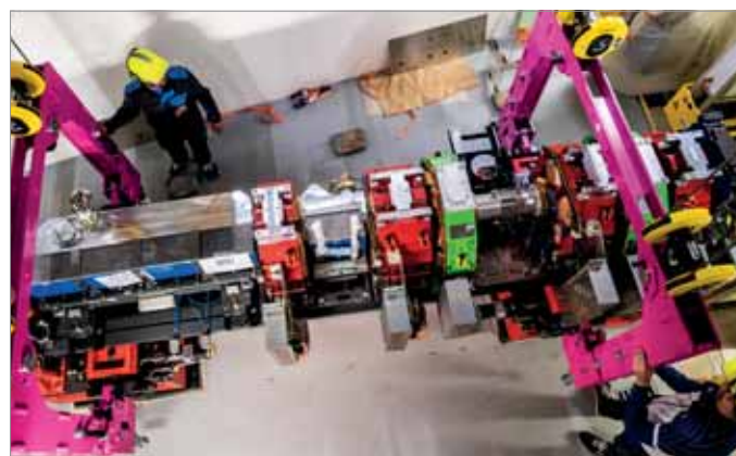
EBS girder installation completed, p14
