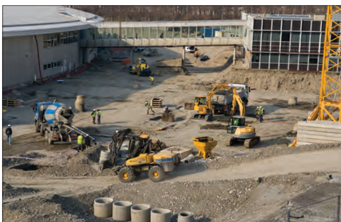
The earth moves: experimental-hall extension takes shape, p14.
