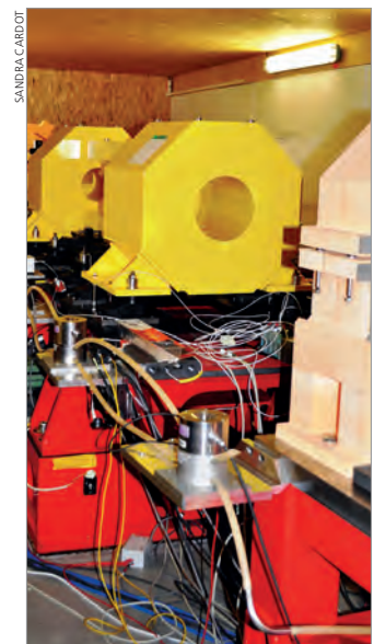
Girder tested for warping in the mock tunnel.
