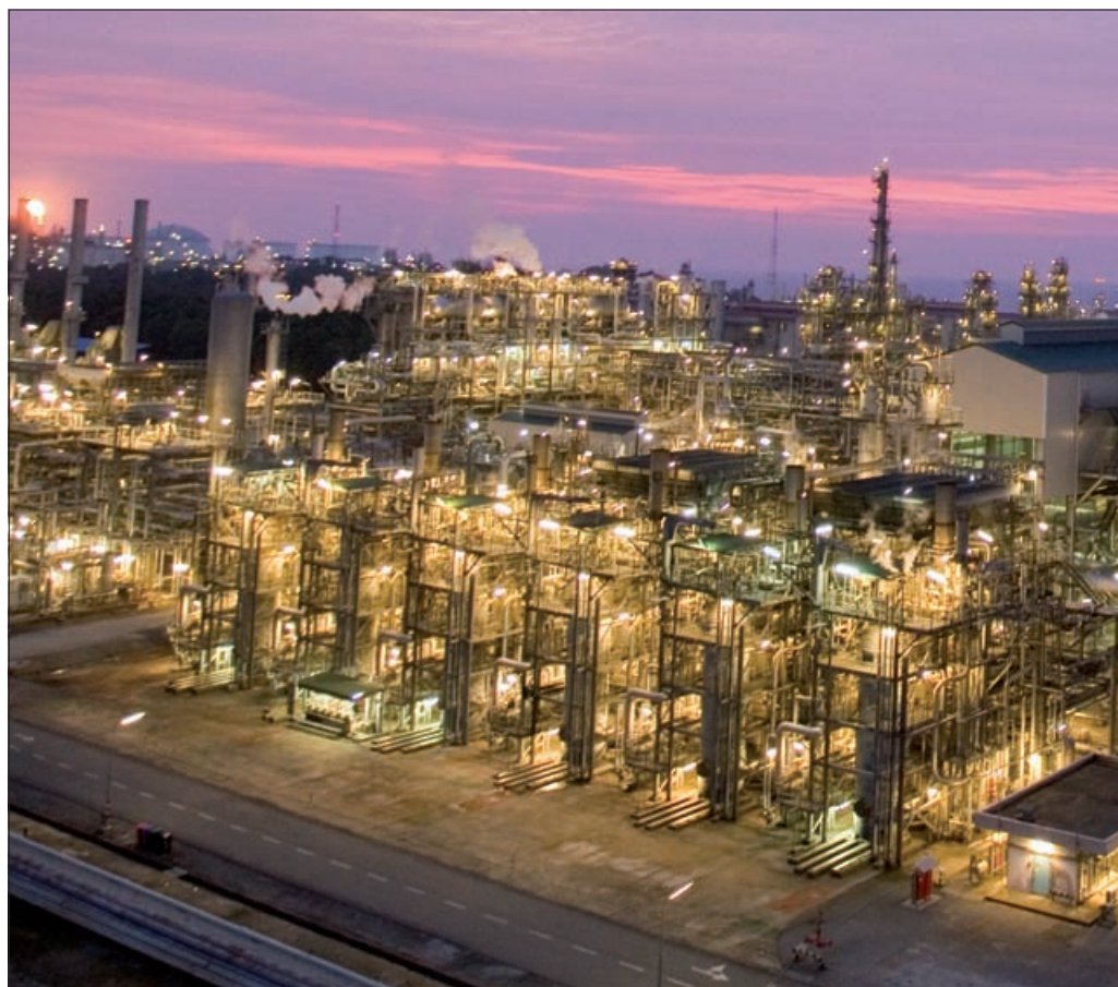
Image of the gas to liquids (GTL) plant of Shell in Malaysia. GTL is a refinery process to convert natural gas or other
