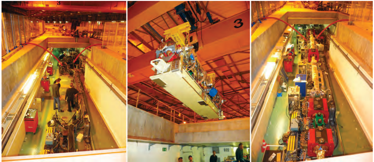
Figure 2.74: Lengthening the straight section in Cell 23 during the 2012 winter shut down.
